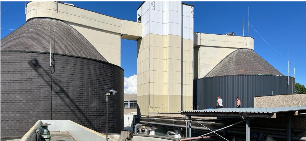
Figure 5-1: The two anaerobic digester tanks at the Wallern WWTP, Austria, May 2024
