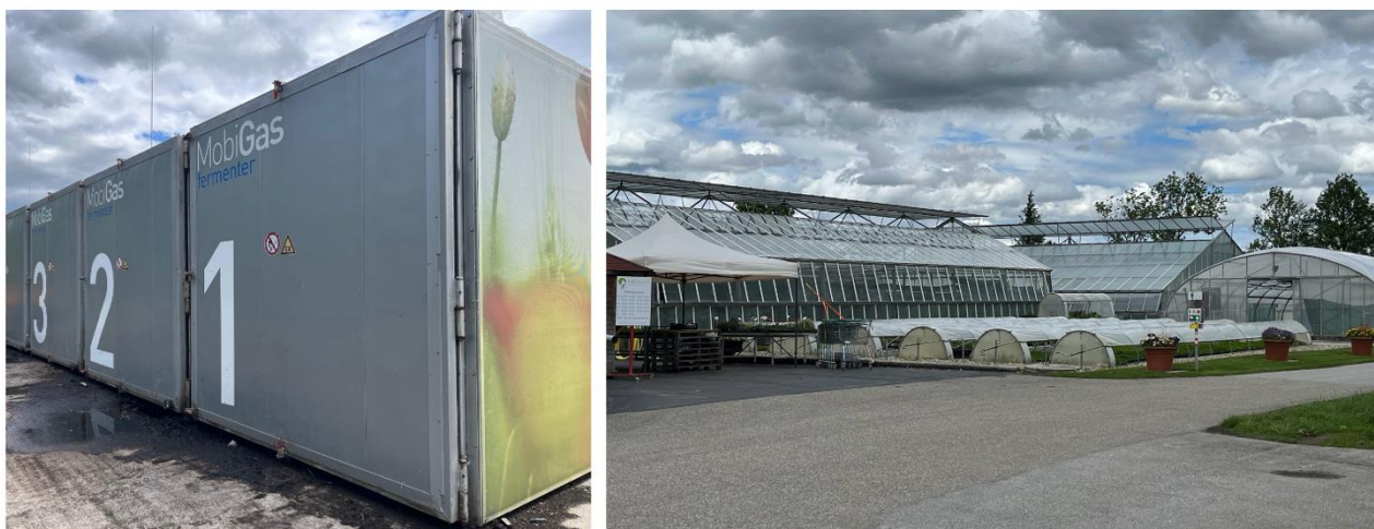
Figure 5-15: Dry AD cells at Drexler Horticulture, Upper Austria. This business grows seedlings for residential and commercial customers and operates the dry AD cells and a compost facility as part of its operations. Compost is used onsite and sold, and biogas provides heat to the greenhouses. May 2024
