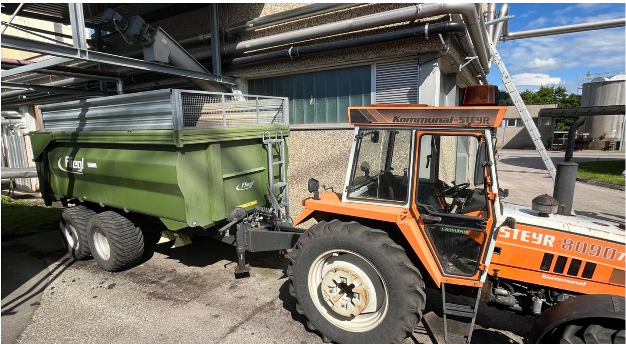
Figure 5-2: Dewatered digestate at the Wallern WWTP being discharged from a screw conveyor into the waiting spreading rig, Austria, May 2024
