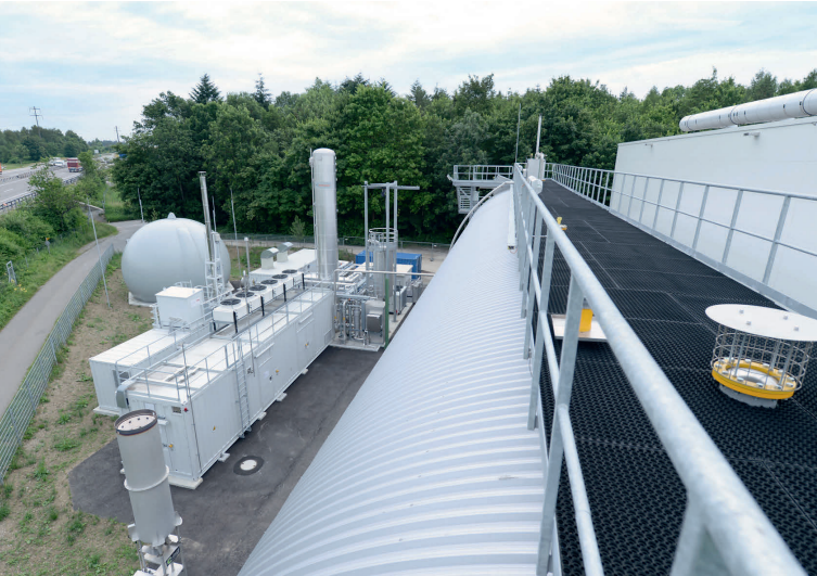
Winterthur: The HZI BioMethan gas treatment plant operates by means of pressureless amine scrubbing
