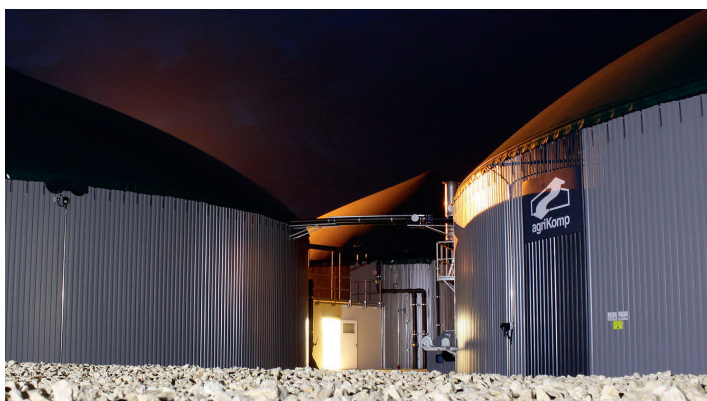
agriPure – Gas-to-Grid Plant System by agriKomp GmbH
