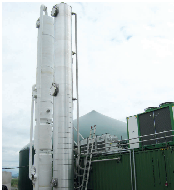
Water scrubbing unit of the Fraser Valley Biogas Plant
