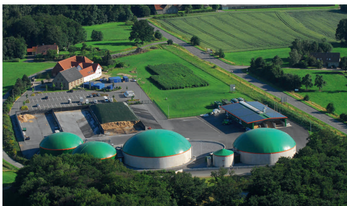
A view on BioConstruct's Headquarter and own operated anaerobic digestion plant
