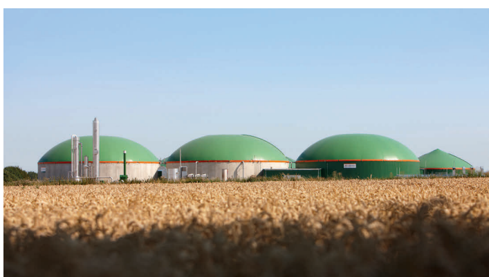
Biogas plant Vettweiß biomethane feed-in plant
