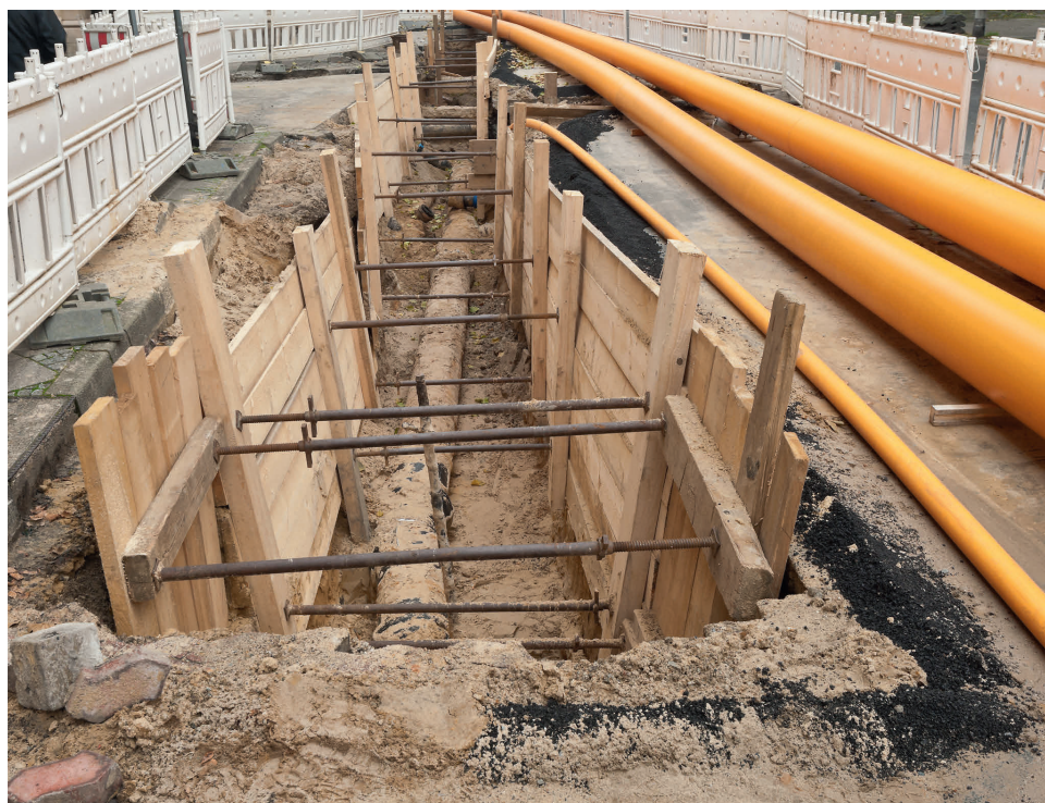
Construction of biomethane pipelines
