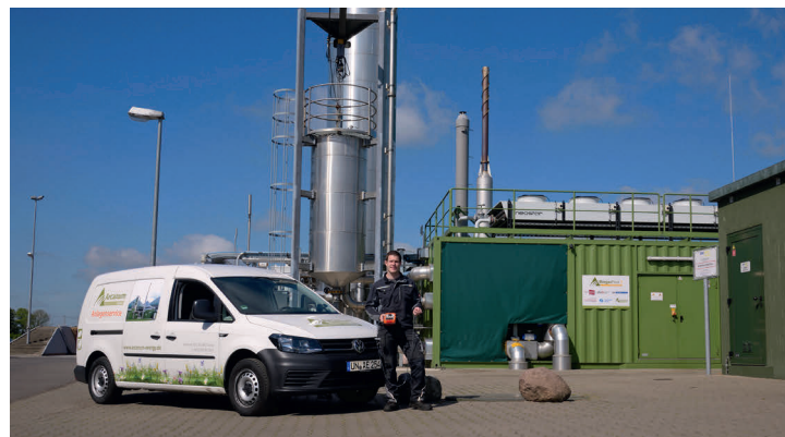
Supplier of project development and plant service
