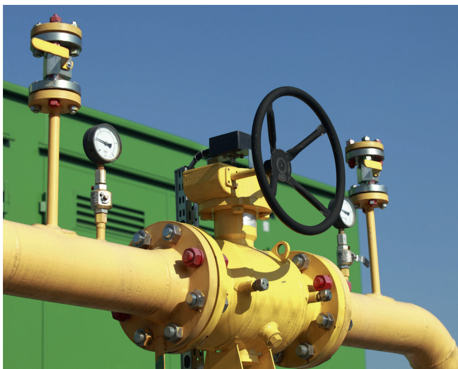
The gas grid access has to be regulated precisely
