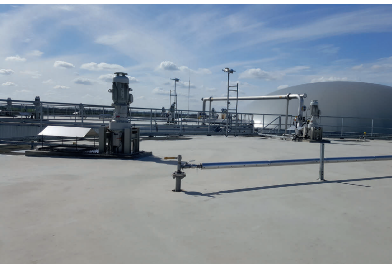
View from digester roof top: High performance mixer drives for stirring up to 16% dry matter. Large-scale gas buffers on post-digesters
