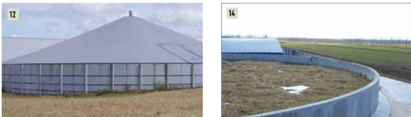
Figure 3: Left - Biofertiliser storage tank covered with gas tight membrane (soft cover). Right - open storage tank with straw on the surface (Seadi et al., 2010).
