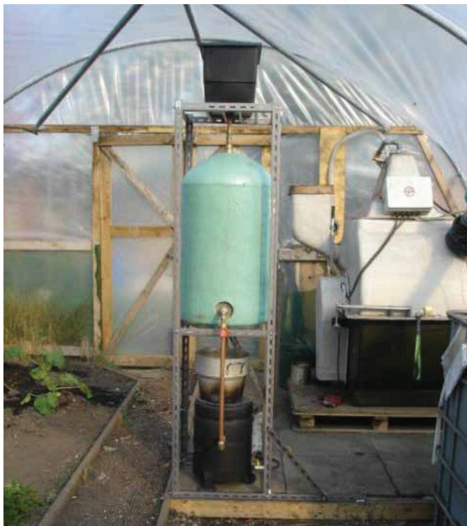
System showing digester in the background with hot water boiler in the foreground.
