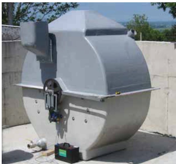
2m 3 biogastronome running on solar PV in process of being installed.
